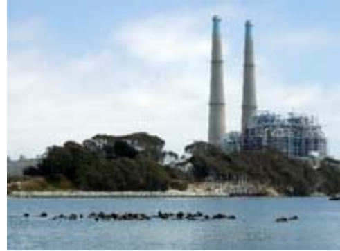
Moss Landing Power Plant. Source: Gerick Bergsma, 2009 Marine Photobank.
